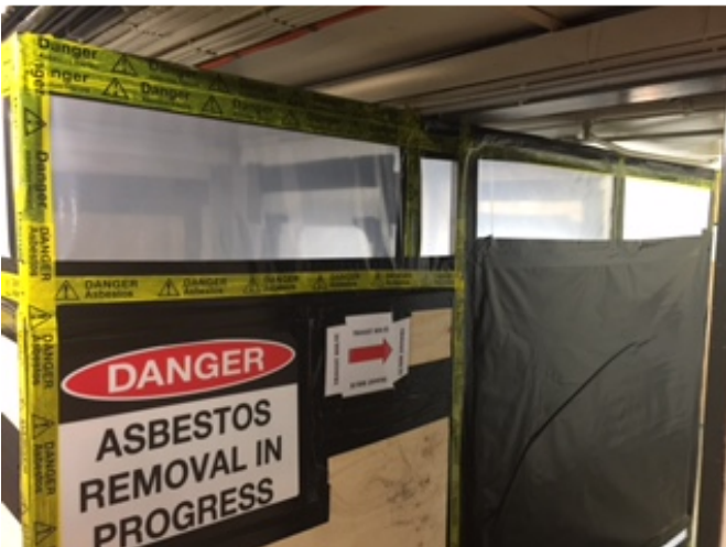
Airlock with signage and timber protection
