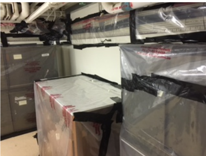
Encapsulation of internal fittings room B6
