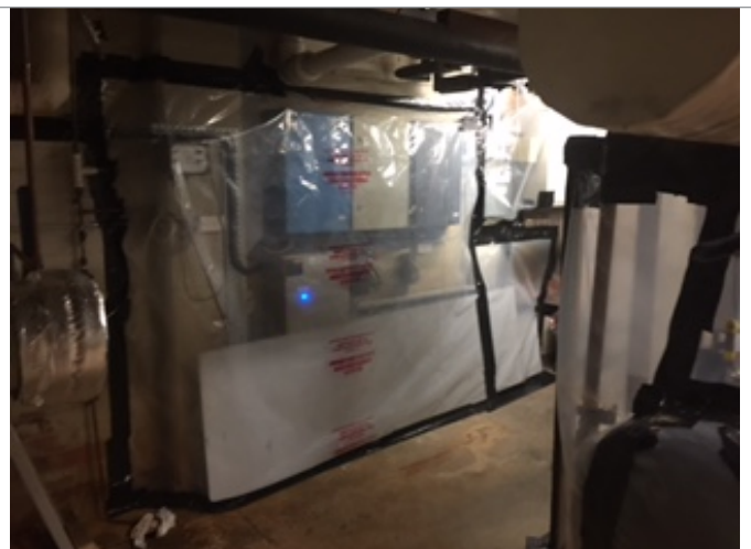
Encapsulation of internal areas in main plant room
