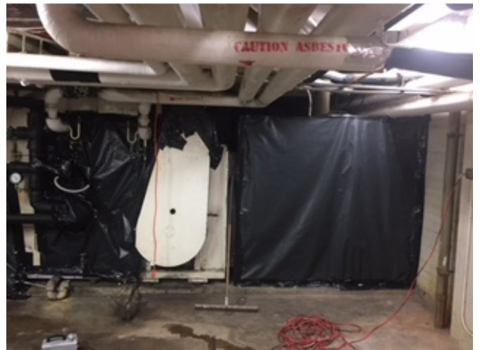
Encapsulation of Air handling unit in main plant room
