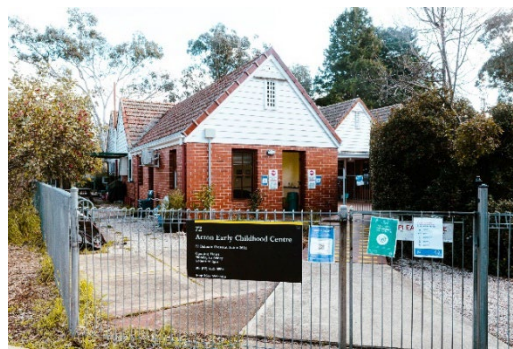
Acton Early Childhood Centre (Building 72)
