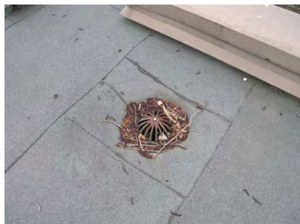
Figure 4.8: The roof of Toad Hall was originally covered with gravel, but has since been overlaid with bituminous roofing material to address recurrent leaks. Expressive rain-heads lead to circular down-pipes that are embedded within the structure.
