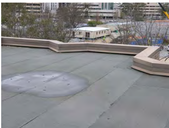
Figure 4.8: The roof of Toad Hall was originally covered with gravel, but has since been overlaid with bituminous roofing material to address recurrent leaks. Expressive rain-heads lead to circular down-pipes that are embedded within the structure.
