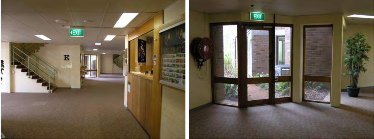
Figure 4.4: The ground floor was originally open and provided hanging racks and easy access for bicycles. The walls have been painted, carpet laid and a false ceiling installed to hide the services. These were substantial alterations to the original design, and include introduced features such as the timber joinery.
