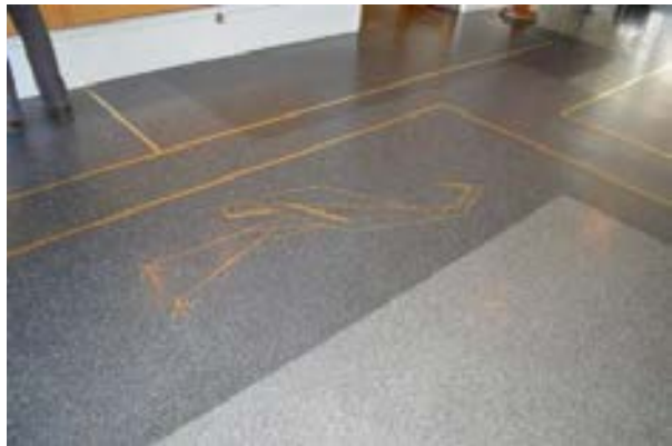
Figure 3.19 Entrance foyer showing brass inlay terrazzo floor designed by Frank Hinder. (Source: GML 2015)
