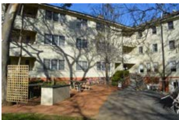
Figure 3.102 Western Annex (R), Fellows Garden and accommodation wing (L). (Source: GML 2015)
