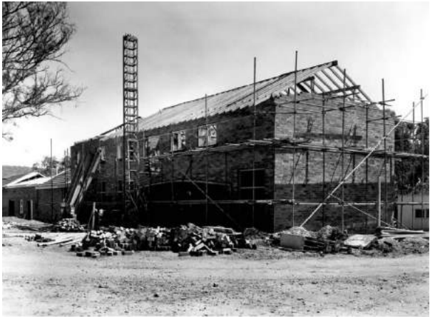
Figure 2.19 Molly Huxley Building under construction 1963. (Source: ANU Archives 2015)
