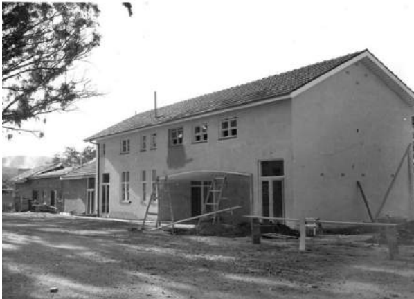
Figure 2.21 Molly Huxley Building under construction 1963. (Source: ANU Archives 2015)
