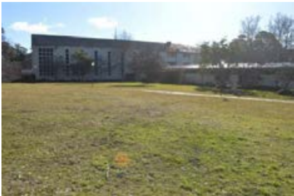
Figure 3.4 View across the southern lawns to the Great Hall. (Source: GML 2015)
