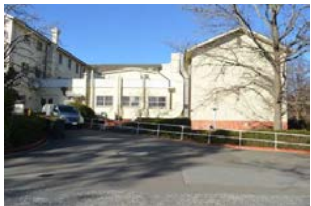
Figure 3.97 Western Annex. (Source: GML 2015)
