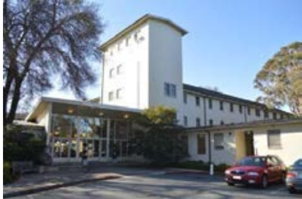
Figure 3.3 The front entrance of University House. (Source: GML 2015)
