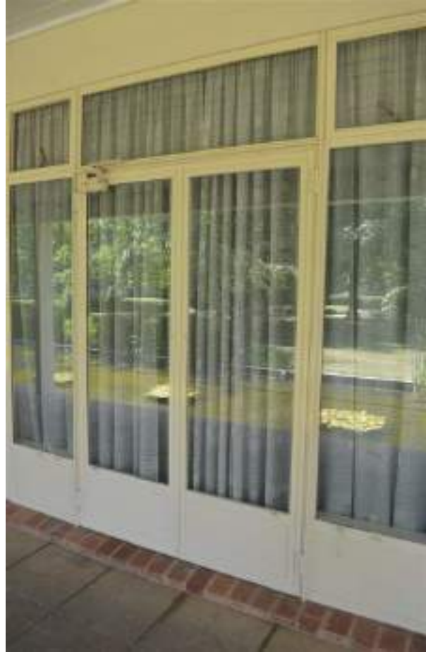
Figure 3.47 Terrace showing the glazing and steel-framed windows and doors of the Common Room. (Source: GML 2015)
