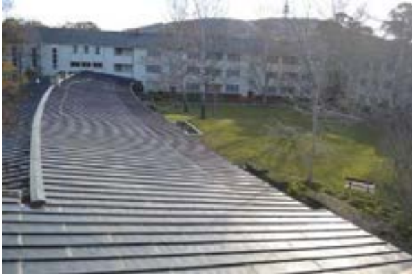
Figure 3.45 Main Block copper-panelled roof and view into courtyard. (Source: GML 2015)
