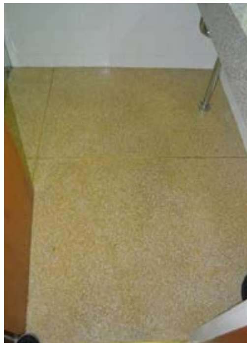
Figure 3.77 Original terrazzo flooring in bathroom. (Source: GML 2015)
