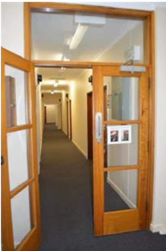
Figure 3.106 Ash timber doors in the Western Annex. (Source: GML 2015)
