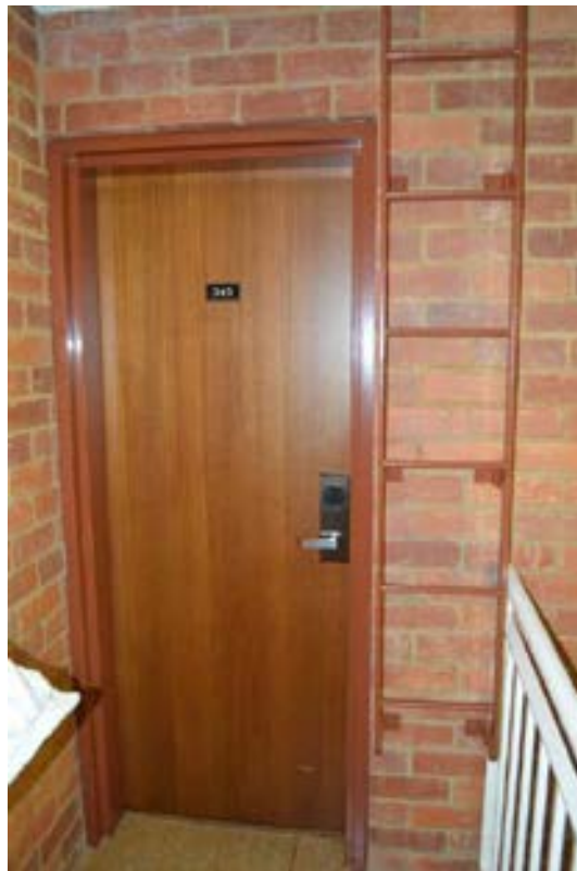
Figure 3.87 Card readers on original doors in the accommodation wing. (Source: GML 2015)
