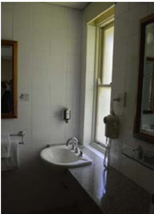
Figure 3.76 Partly modified bathroom in accommodation wing. (Source: GML 2015)
