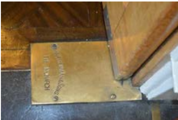
Figure 3.52 Original brass floorplate housing door bearings. (Source: GML 2015)
