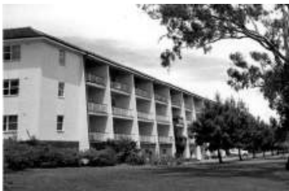
Figure 6: View of the northern façade of University House 1963, including landscaping. (Source: ANU Archives)
