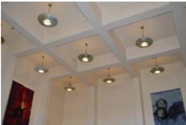
Figure 3.33 'Egg-crate' ceiling in hall foyer and original design lamps. (Source: GML 2015)
