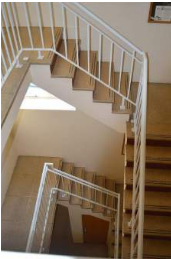
Figure 3.68 Eastern annex stair well. (Source: GML 2015)
