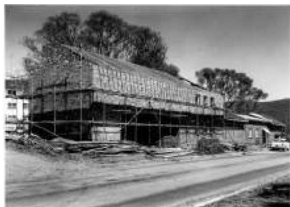
Figure 7: Construction of the Molly Huxley Building in 1964. (Source: ANU Archives)
