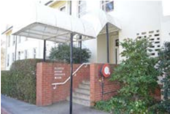
Figure 3.113 Entry to Scarth and Stanner Rooms, south side of western annex. (Source: GML 2015)
