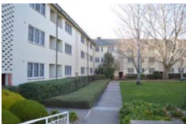
Figure 3.10 Courtyard perimeter path and western side accommodation wing. (Source: GML 2015)
