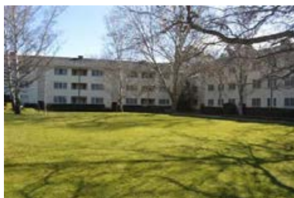
Figure 3.11 Courtyard and accommodation wing. (Source: GML 2015)
