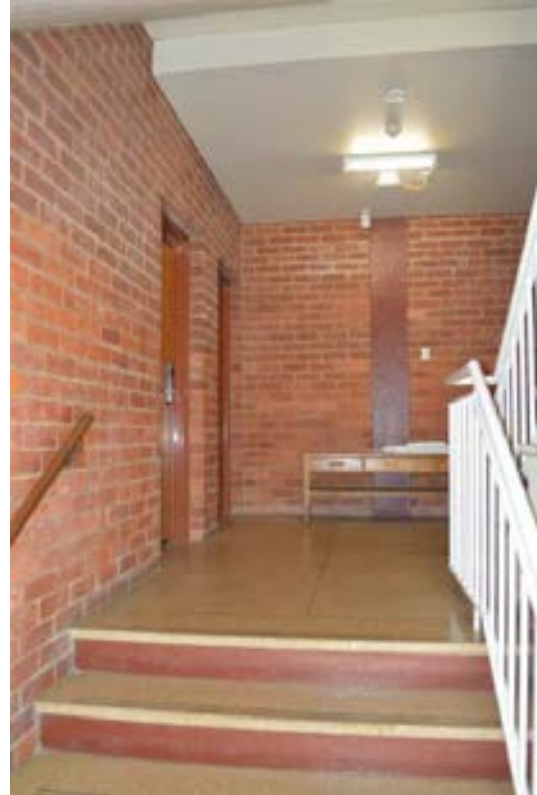
Figure 3.89 Red brick in stairwells with terrazzo stair treads, accommodation wing. (Source: GML 2015)
