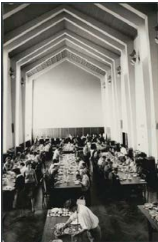
Figure 2.11 The Great Hall, University House c1964 (Source: National Library of Australia 2015)
