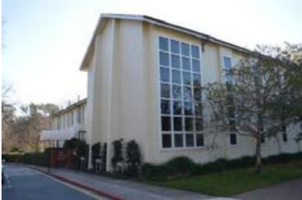
Figure 3.2 The Great Hall at the front of University House. (Source: GML 2015)
