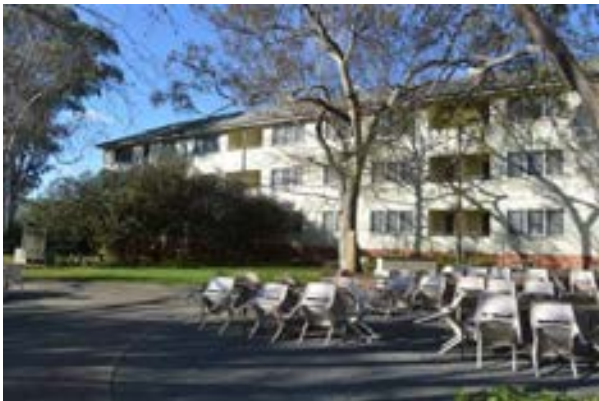
Figure 3.56 West side of the accommodation wing with Fellows Garden in the foreground. (Source: GML 2015)
