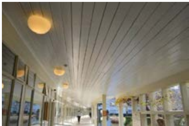
Figure 3.17 Timber-lined roof of terrace. (Source: GML 2015)
