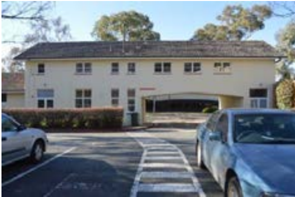
Figure 3.137 Molly Huxley Building. (Source: GML 2015)
