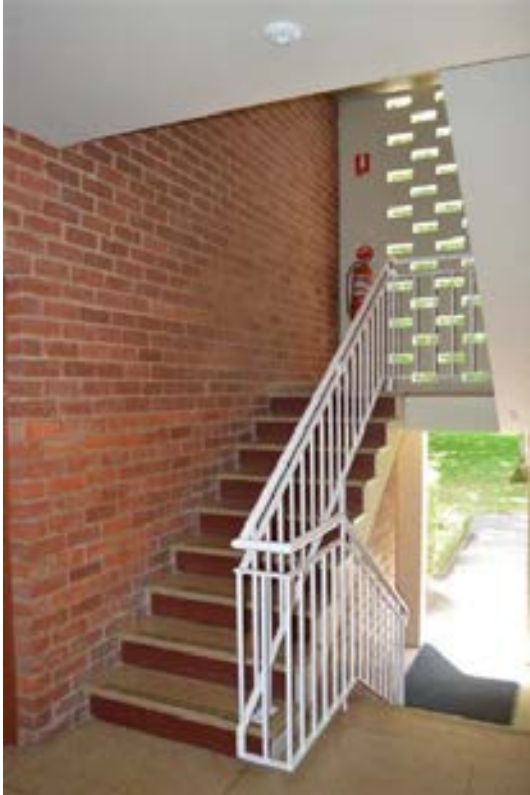
Figure 3.88 Red brick in stairwells with terrazzo stair treads, accommodation wing (Source: GML 2015)
