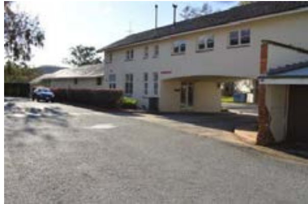
Figure 3.138 Molly Huxley Building. (Source: GML 2015)
