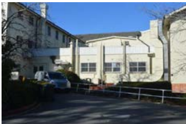
Figure 3.98 Western Annex, two-story kitchen section in centre. (Source: GML 2015)
