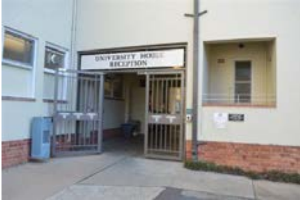
Figure 3.66 Entrance to terrace and University House from northeast carpark. (Source: GML 2015)
