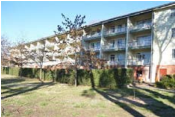
Figure 3.58 North side of the accommodation wing. (Source: GML 2015)
