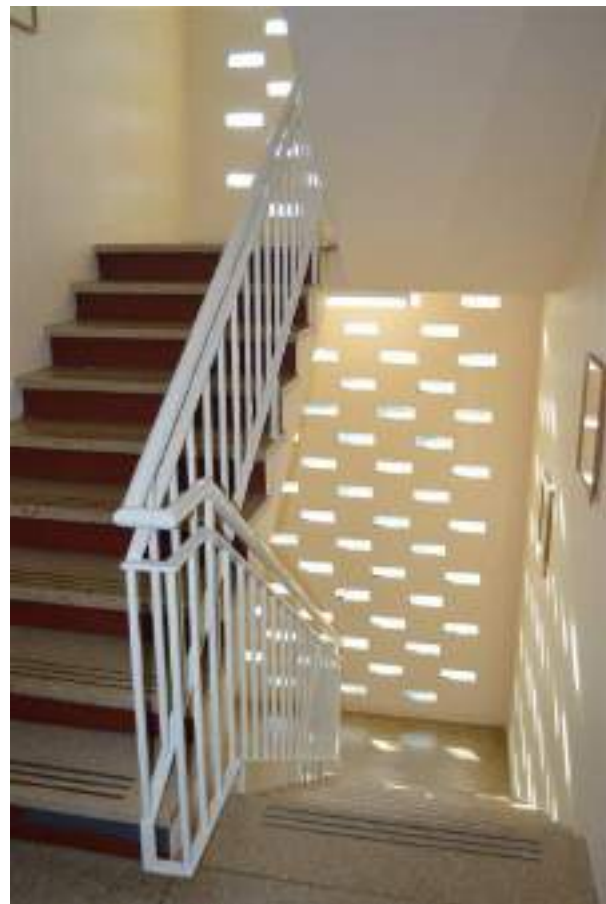
Figure 3.69 Eastern annex stair well (hit and miss brickwork feature). (Source: GML 2015)
