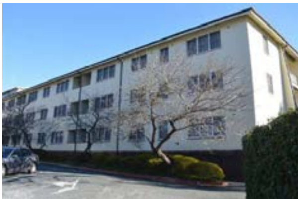
Figure 3.60 East side of the accommodation wing. (Source: GML 2015)
