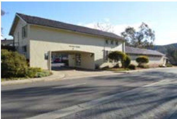
Figure 3.139 Molly Huxley Building, view from northeast. (Source: GML 2015)
