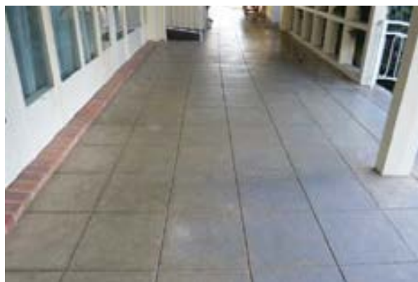
Figure 3.44 Original terrace concrete flooring. (Source: GML 2015)
