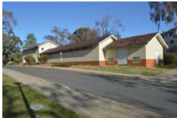
Figure 3.140 Molly Huxley Building, view from northwest. (Source: GML 2015)
