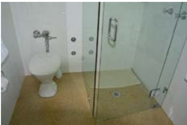
Figure 3.78 Partly modified bathroom in accommodation wing. (Source: GML 2015)
