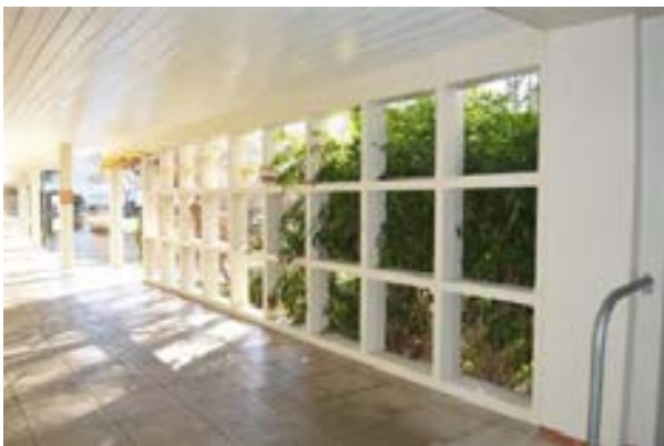
Figure 3.16 Terrace just outside the foyer showing concrete lattice screen. (Source: GML 2015)
