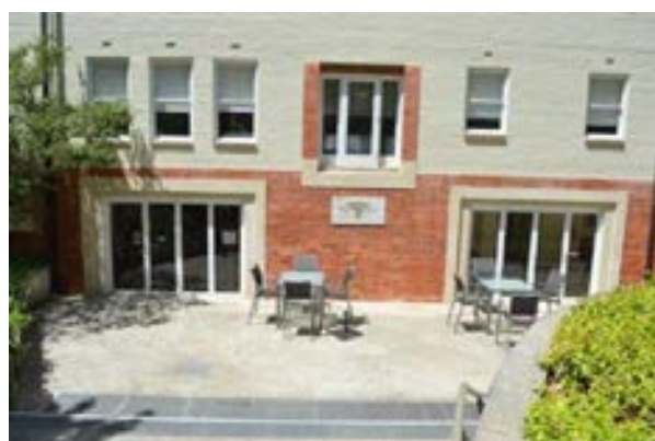
Figure 3.103 Western Annex looking down to lower level entry to Fellows Bar with contemporary fitout, doors and courtyard upgrade. (Source: GML 2015)
