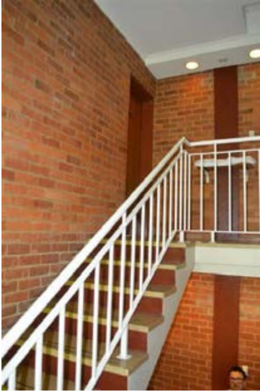
Figure 3.84 Exposed red brick in stairwells with terrazzo stair treads, accommodation wing. (Source: GML 2015)
