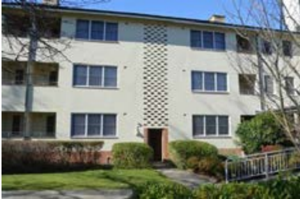
Figure 3.54 Accommodation wing—entry into stairwell and 'hit-and-miss' brickwork. (Source: GML 2015)
