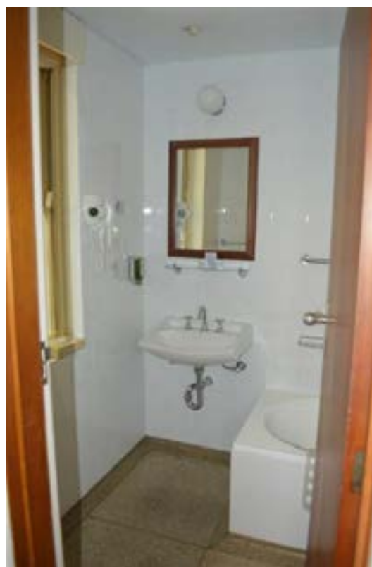
Figure 3.83 Partly modified bathroom in accommodation wing. (Source: GML 2015)
