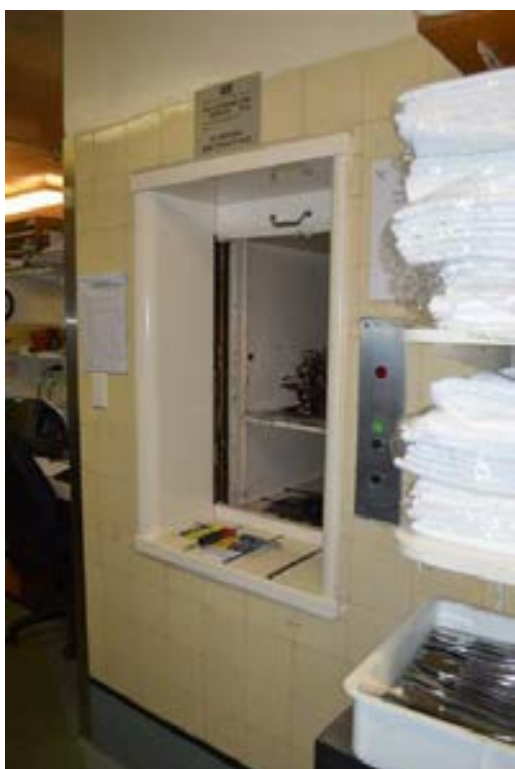
Figure 3.123 Dumb waiter in the servery. (Source: GML 2015)
