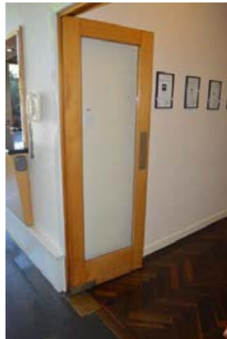
Figure 3.53 Timber-framed door to central corridor of the main block. (Source: GML 2015)
